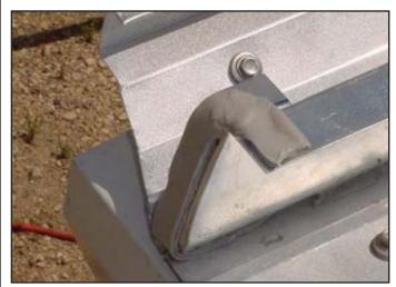
Photo 3: Rake Zee modified at Eave Trim Photo 4: Rake Zee modified at Gutter
