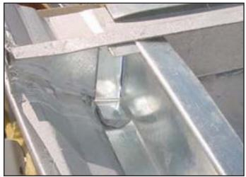
**Photo 1:** Rake Zee modified at End Dam
