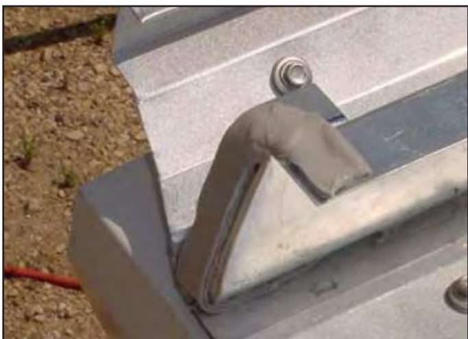
Photo 3: Rake Zee modified at Eave Trim
