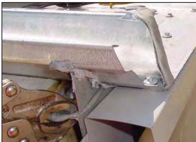
Photo 2: Rake Zee modified at Eave Trim
