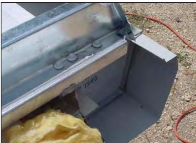
Photo 4: Rake Zee modified at Gutter
